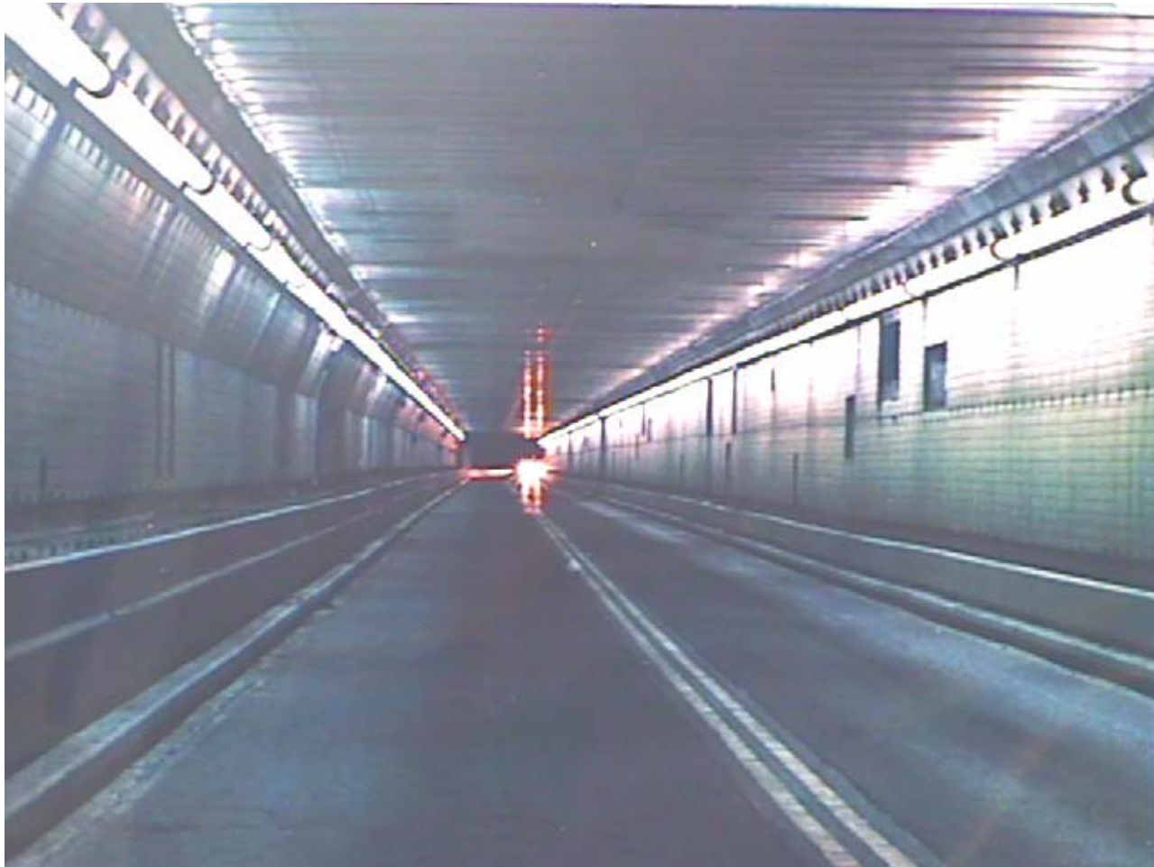
Light Guide Illumination of Boston's Callahan Tunnel
